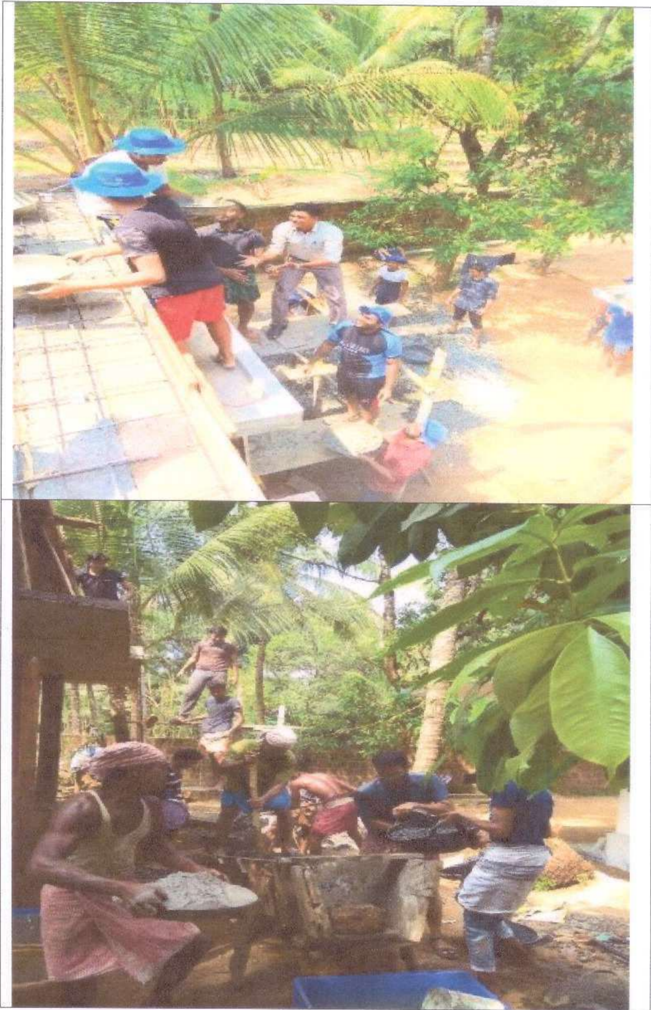
At the Construction Site
