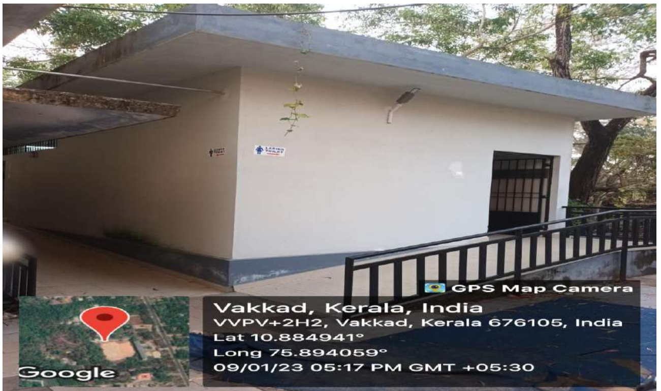
New toilet block
